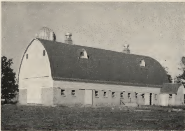
Typical Gothic roof barn with concrete masonry walls up to mow floor.
